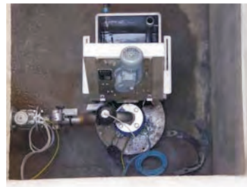
Oil skimmer model 2H for groundwater remediation
